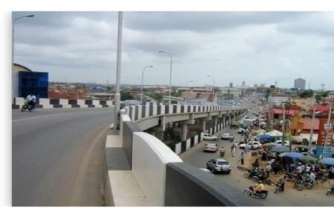
New Bridge at Mokola
