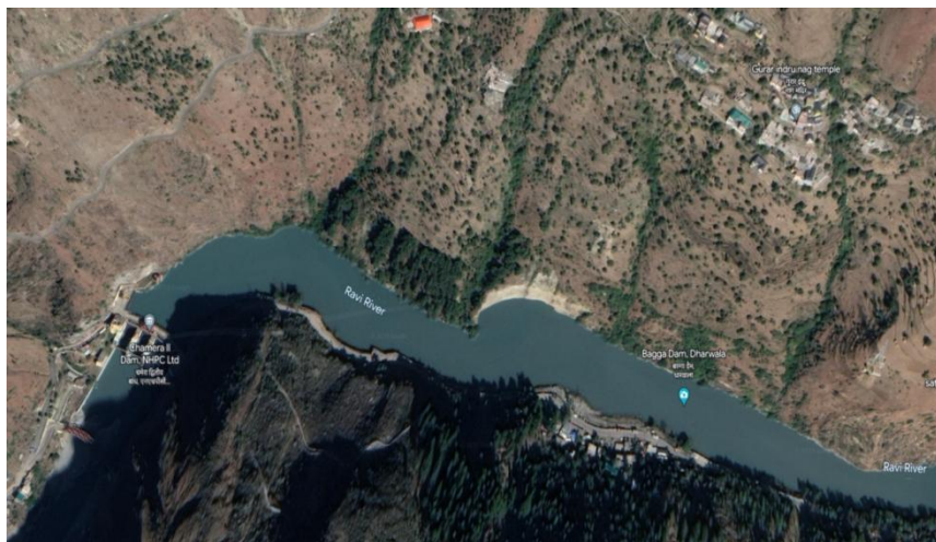
Fig: Pic of Chamera Dam -II
